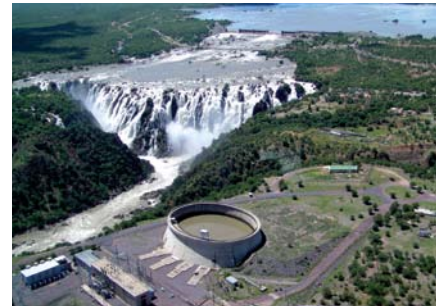
Ruacana hydro Station - Namibia
